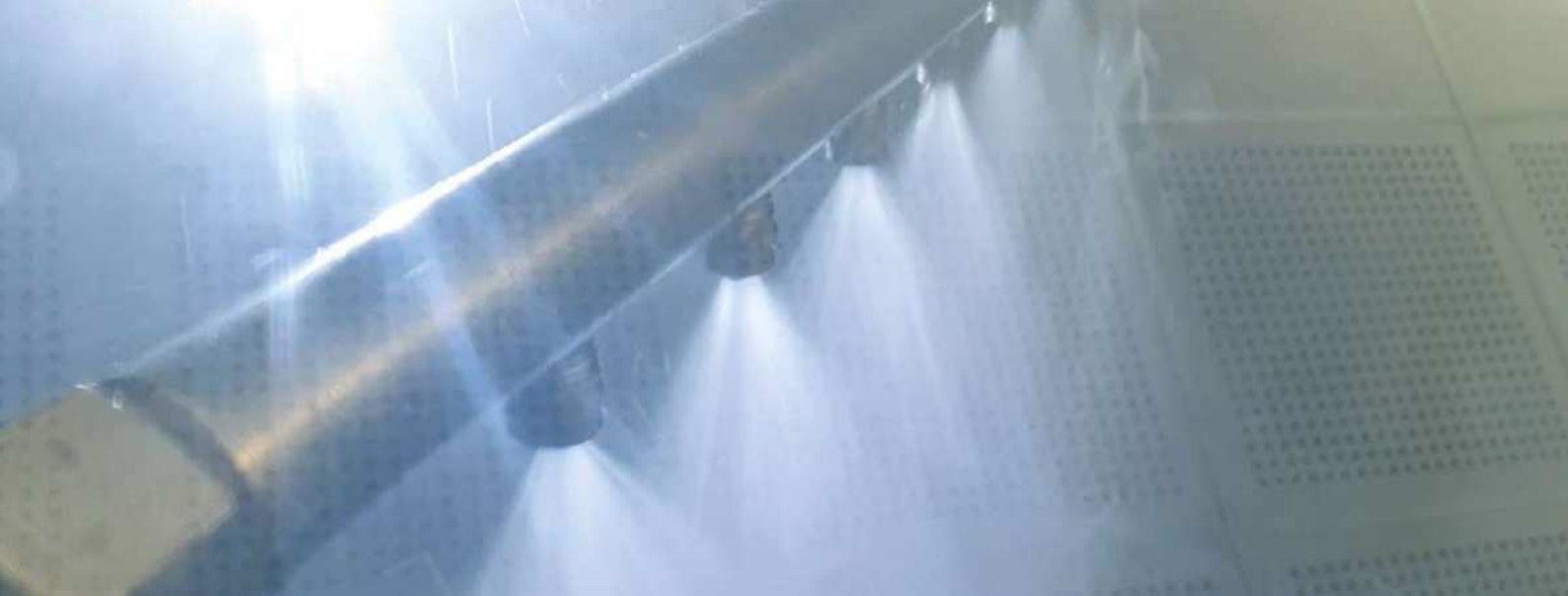
Mechanical cleaning in the HTW
