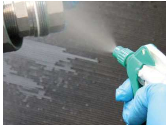
Spray on GS 200 – remove sealant
